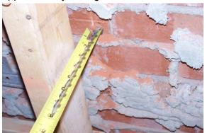
STEP 2- Select a Stitch-Tie helical anchor equal to the distance from the stud face to the to the brick and install per Stitch-Tie installation requirements.
