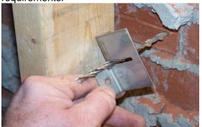
STEP 3) Attach Façade-Tie Bracket to the Stitch-tie anchor.
