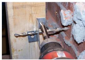
STEP 4- Attach the Façade-Tie Bracket to the stud with the supplied hardware
