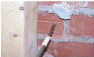
STEP 1- Drill 1/4" hole through the sheathing approximately 1/4"-3/4" from the stud face (parallel with mounting face) into brick or joint approximately 2" or greater.
